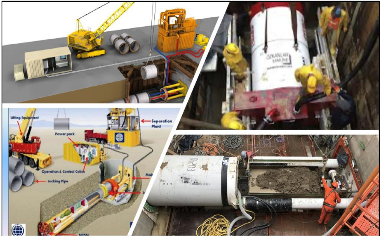
Figure 5.18: Typical micro tunnelling set ups and equipment
