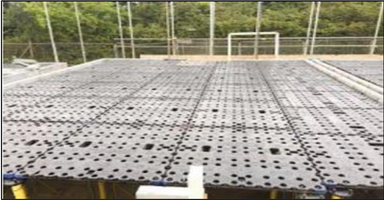
Figure 5.32: Steel crash deck
